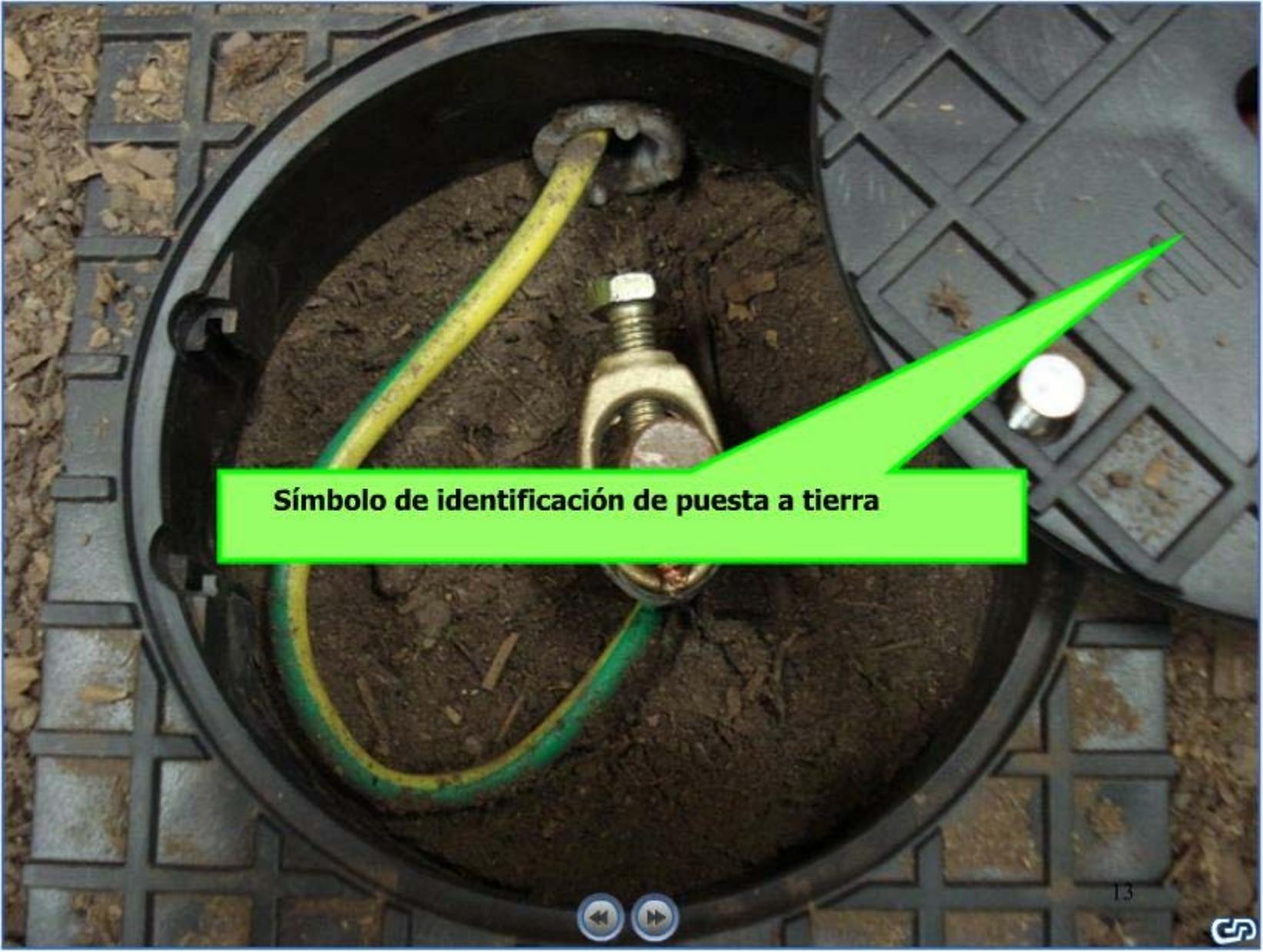
A photograph of an open manhole with a metal grate. Inside, a yellow and green cable is connected to a metal ground terminal. A green arrow points from a text box to the terminal. The text box contains the text "Símbolo de identificación de puesta a tierra".
